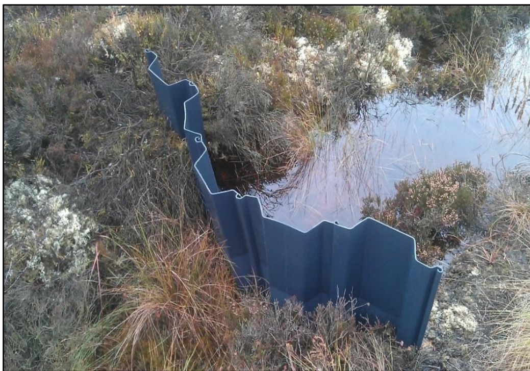
Plate 6. An example of a recycled plastic dam used to block functioning drains on a raised bog site.
